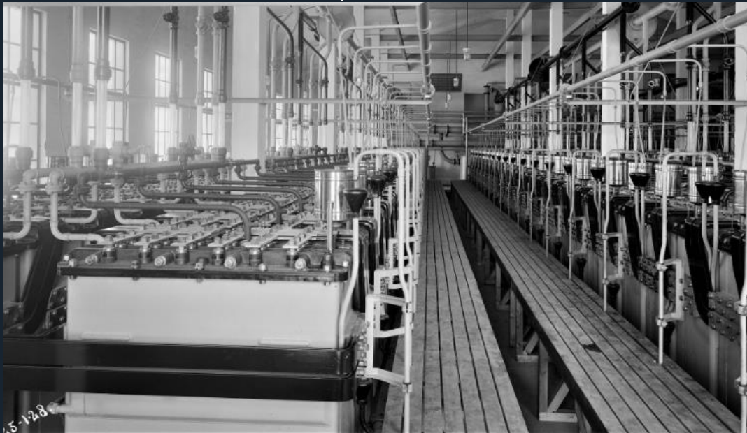
5MW test plant, Notodden, Norway ~1928 (Holmboe-cellen, monopolar)
